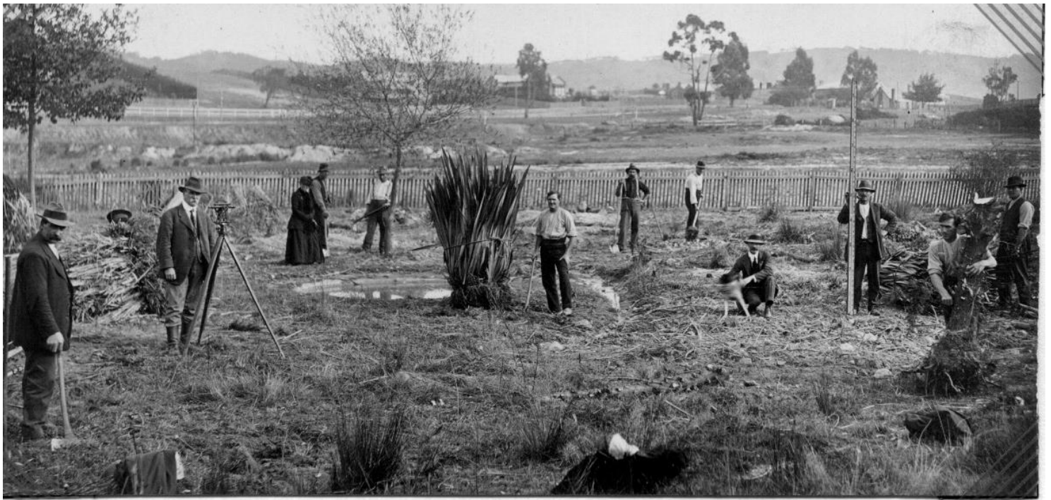
Surveying the site for the new sports ground
